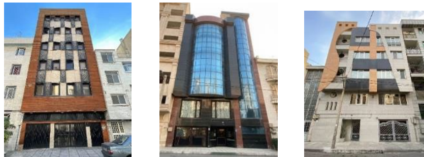
Figure 2. Form in the façade of a residential building (Author, 2026).
