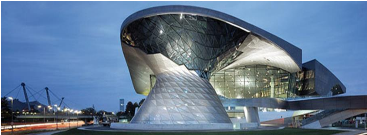
Fig 1 Exterior view to the BMW Welt Munich, Germany (Source: https://www.e-architect.co.uk )
