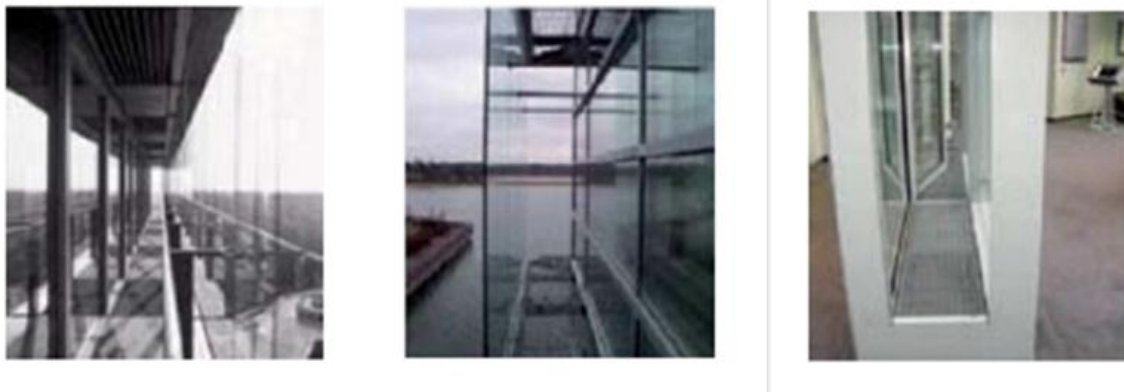
Fig 1 From left to right: the outer shell, the airspace, the inner shell, a double skin façade (Zolfaghari et al., 2013)
