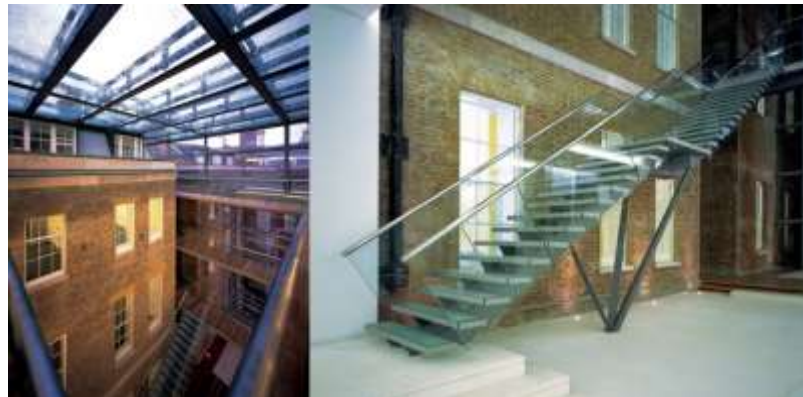
Fig 10 Conservation a historic building in London in a cover of modern structure ( http://www.hok.com/design/service/renovation-restoration/cabinet-office-22-26-whitehall )
